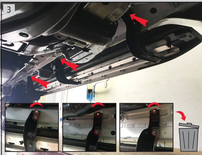
Remove 6 bolts and dispose left step
